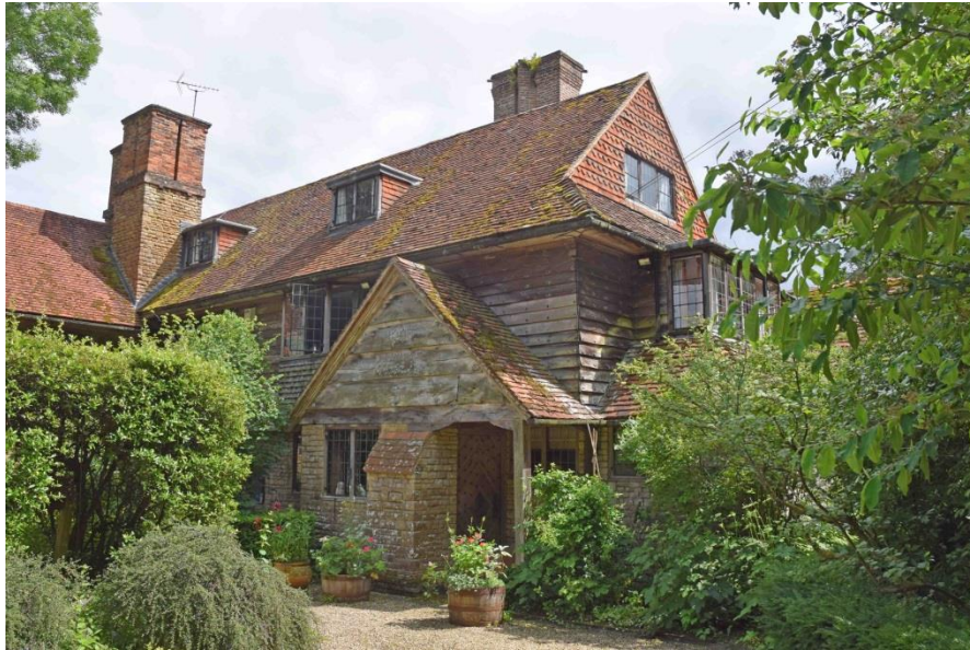
Porch to the house on the south side of Caroe wing
